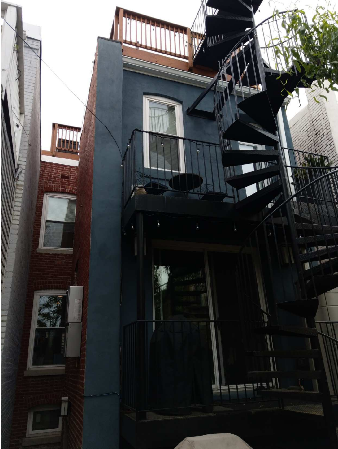
Existing Rear Elevation (From inside yard)
